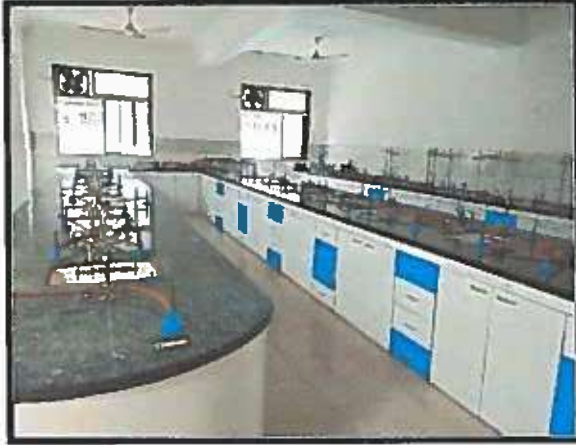
Exhaust Fan in Chemical Laboratory and good ceiling height
